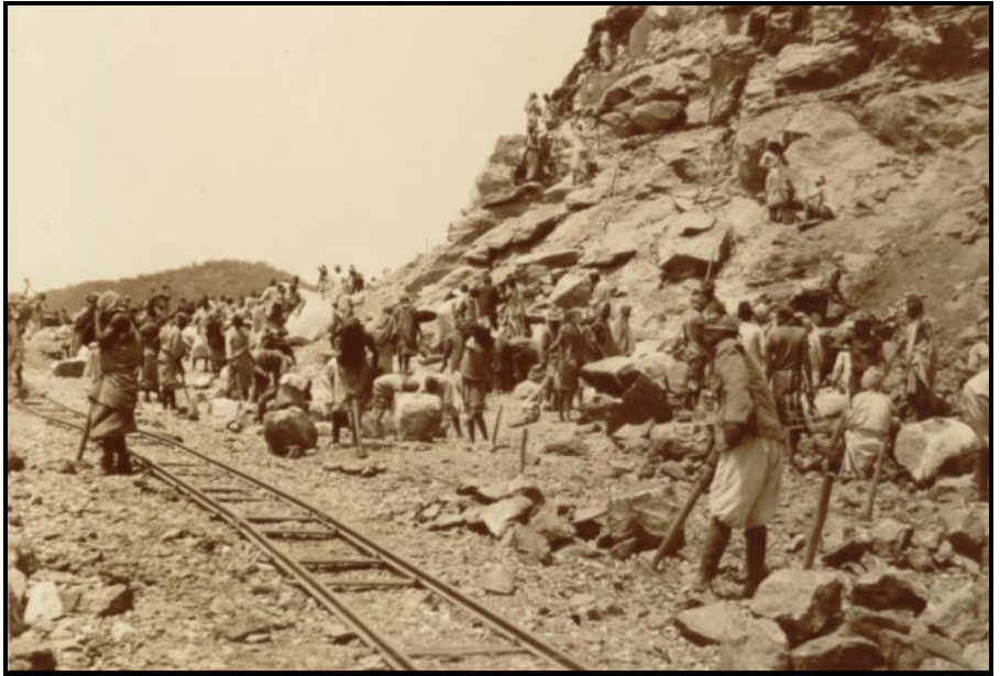
Creating the infrastructure of empire: African workers building the German East African railroad, circa 1905-1907.
